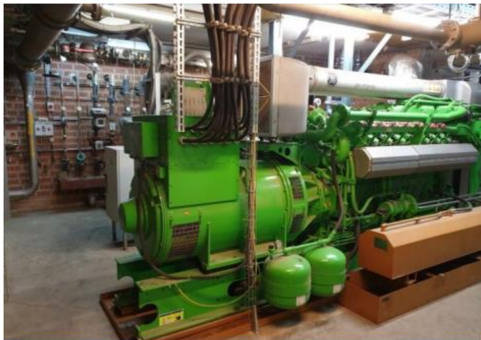
Figure 10: A typical CHP unit powered by biogas.
